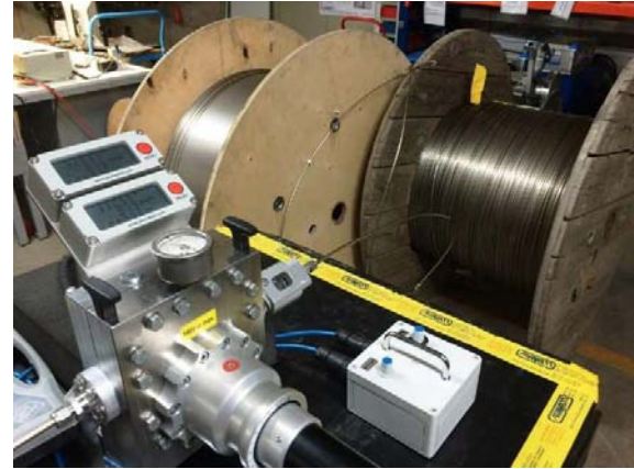
Figure 8. Floating 485 \mu\text{m} fiber into 5.0/4.5 m welded steel tube of 5.2 km long, with alcohol. Big pressure tank used. 2 km was installed with 100 bar alcohol coming out at end of tube. Fiber speed 13 m/min.
